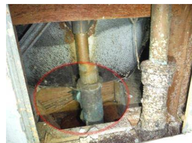
Leaking tub drain
