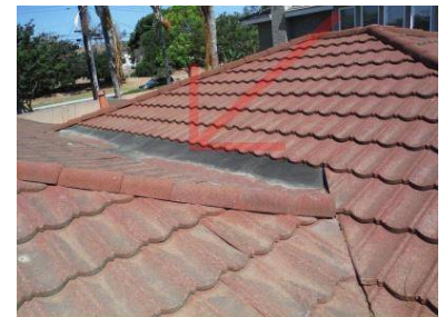
This area will need periodic sealing
