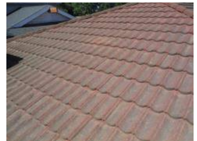
This area will need periodic sealing
